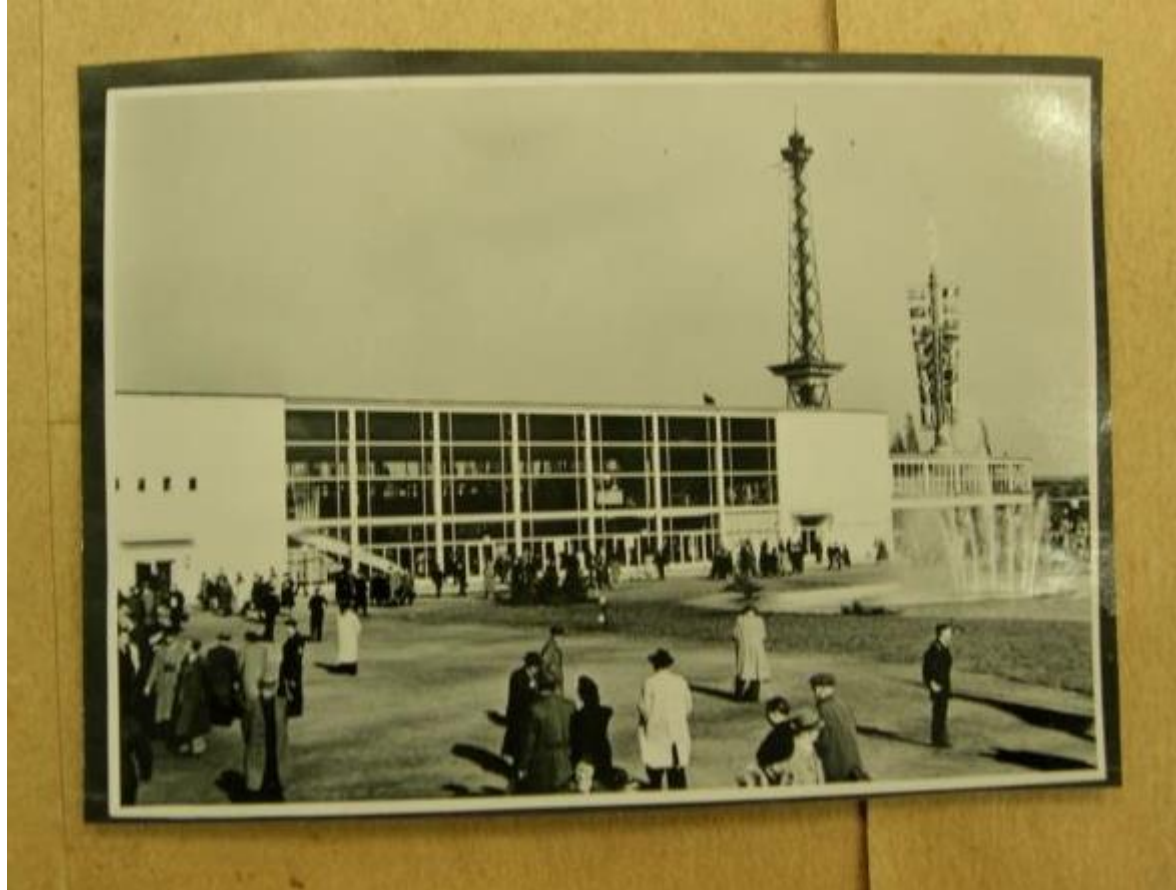
Germany's Pavilion: The Marshall House
