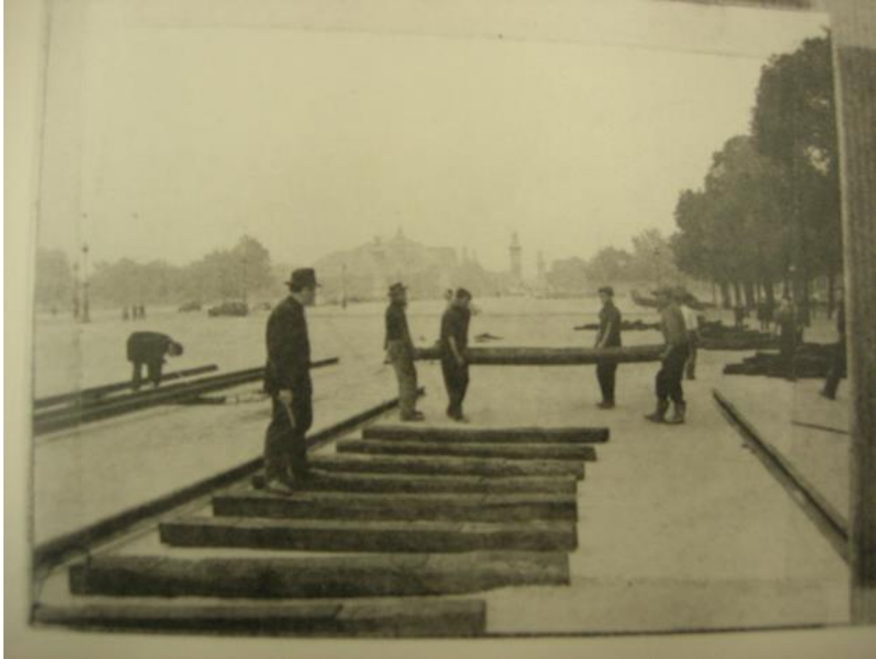
Europe Train, Laying the Tracks, 1951 Paris
