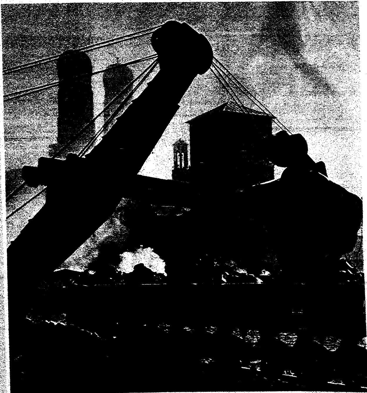
Modern technology helped clear away ruins made by modern destruction. Here a steam-shovel removes rubble in Munich in 1947. In the background one can see silhouetted the famous towers of the Frauenkirche whose exterior has been reconstructed. This cathedral is the symbol of Munich — a well-loved landmark which can be seen for miles around the city
